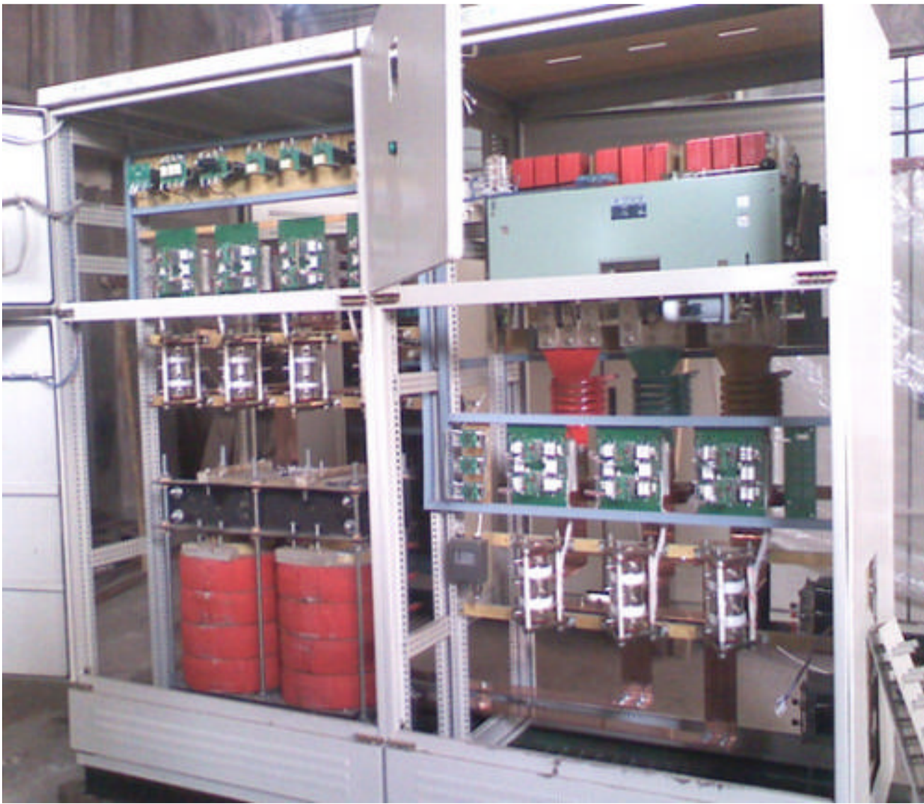
Fig.3: 800kW MFPS with TECHSEM Capsule Devices
